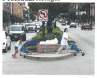
Pedestrian refuges are typically constructed near intersections or in between lanes of traffic to decrease the crossing distance for pedestrians, or to decrease the width of the roadway.
