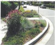
Curb extensions are typically used to decrease the walking distance for pedestrians crossing a roadway. At a pedestrian crossing, the curb is extended closer to the centerline of the street.
