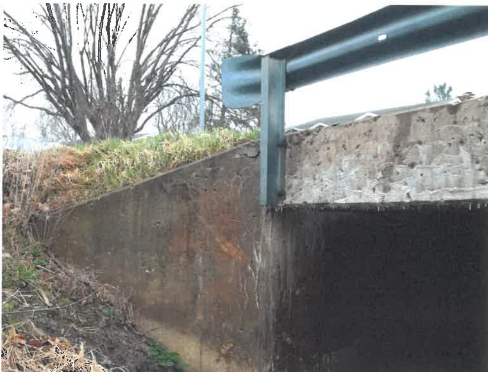
Crazing and leacate noted in the upper slab
