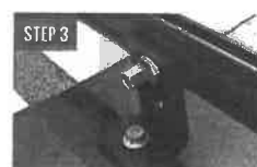
ATTACH L-FOOT TO RAIL
