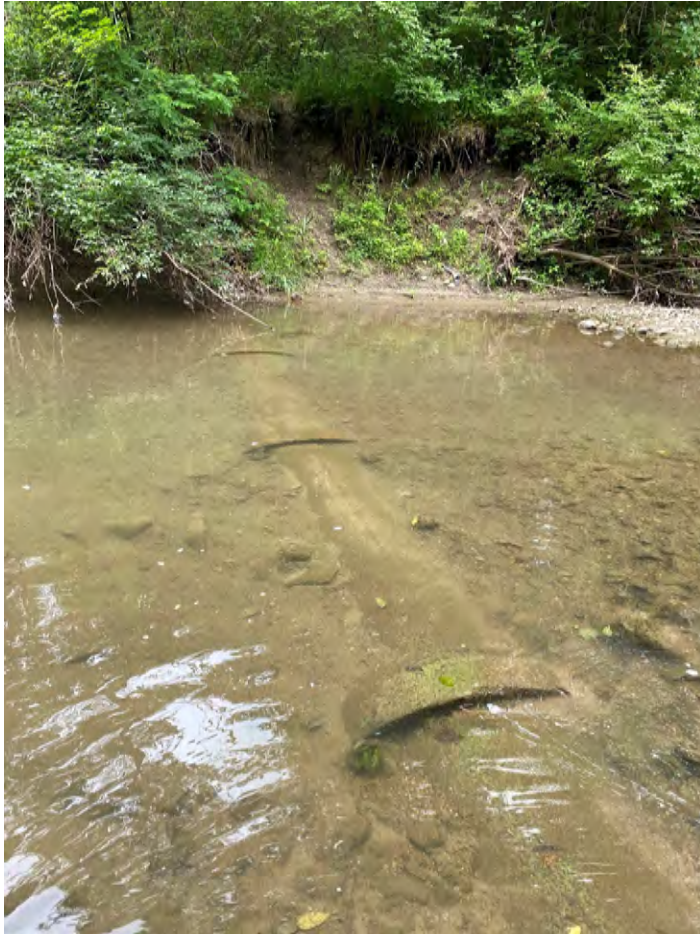
Existing trunk sewer pipe & joint exposed – west Farm Creek bank
