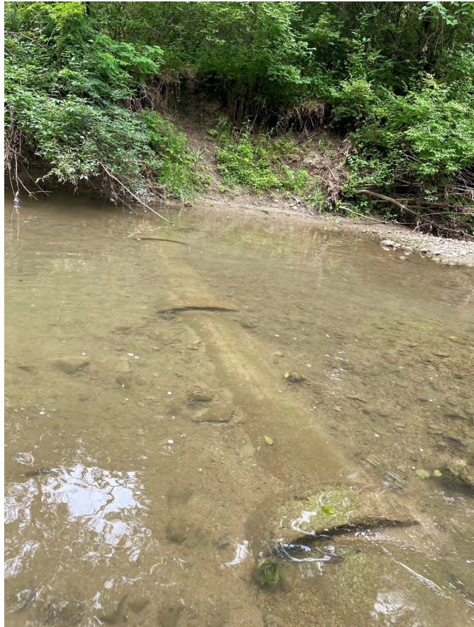
Existing trunk sewer pipe & joints exposed
