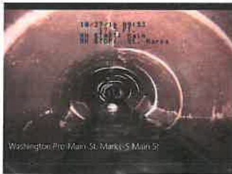
Video of pipe needing lining
